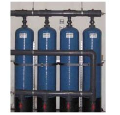
The full weight of the piping and valves must be supported by unistrut, pipe hangers or other means. The tank connections can not support the weight of the piping. This photo from a multitank system insallation shows properly supported piping.
